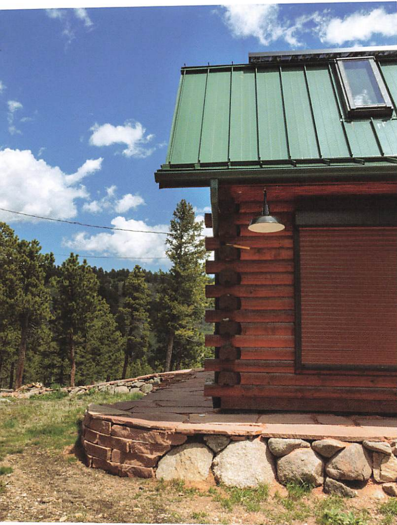
Bottom: A metal roof and noncombustible exterior window coverings add layers of protection against wildfire, in addition to the well-maintained defensible space that surrounds this home. Photo: Wildfire Partners
