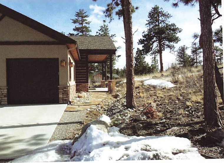
Top left: Hardening your home can include choosing noncombustible building materials like stucco paired with a stone facade. This house near Salida shows you don't have to sacrifice curb appeal to reduce the ignitability of your house. Photo: CSFS
